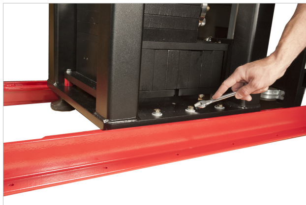
FIGURE 3-8 Removing the cross braces
